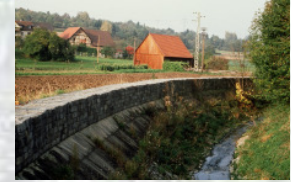
No flood retention possible
